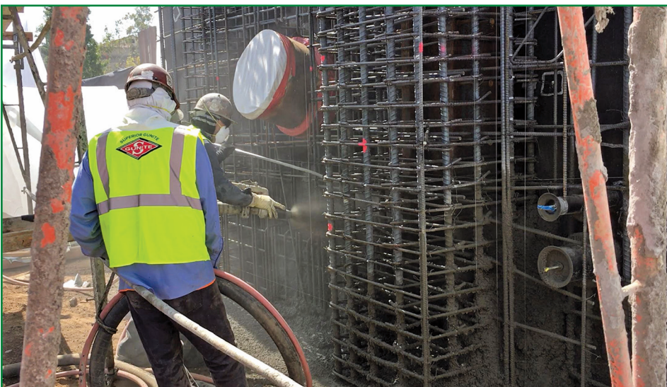
Figure 6 – Observations of the placement of shotcrete.
